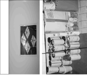
Delay to decay room for radioactive waste
